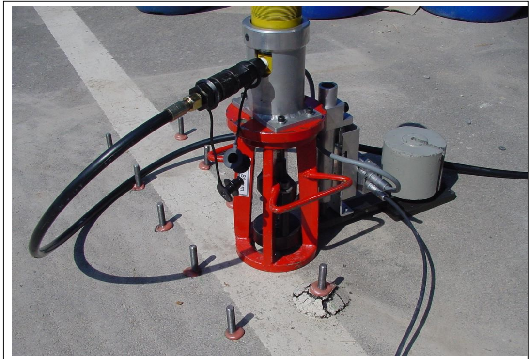
Fig. 1: Tensile testing of HAS M12 anchor rods fastened with Hilti HIT-RE 500 injection adhesive in asphalt base material using the Minipull test equipment.
