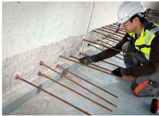
b) Slab-to-wall connection
