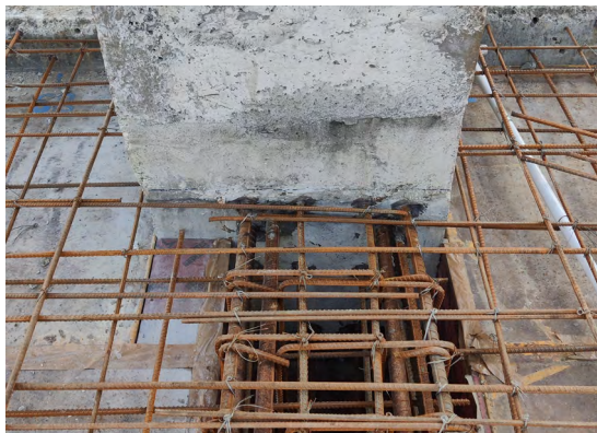
d) Beam-to-column connection
