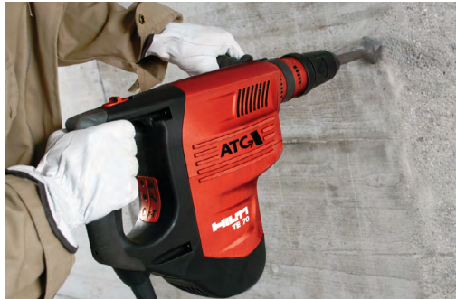
b) Surface roughening using brushing tool
