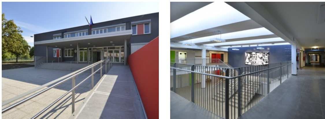
a) Exterior View
