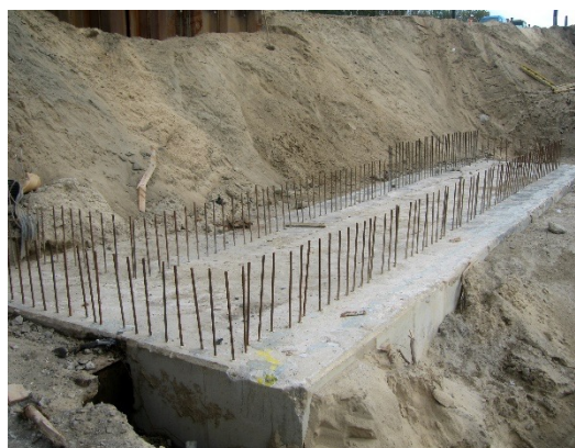
c) Abutment structure with post-installed rebars
