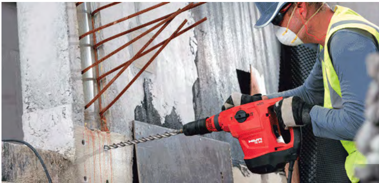
Fig. 9.4: Hammer drilling (HD) tools
