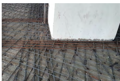
c) Slab strengthening
