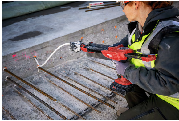
b) Extension hose for adhesive mortar injection
