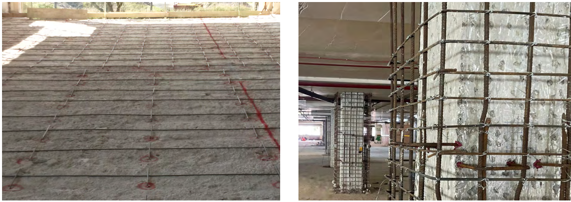
g) Slab shear-friction overlay
