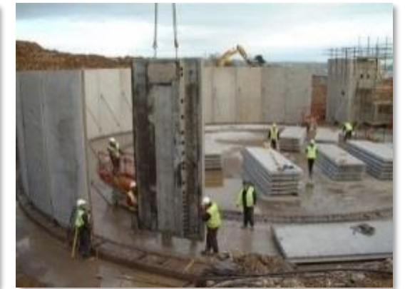
Pre-stressed water tank
