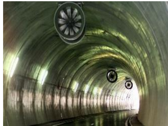
Pre-stressed concrete lining of tunnel
