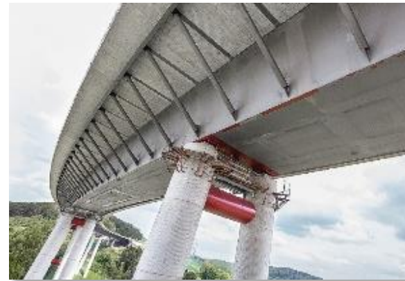
Pre-stressed pile/slab of bridge
