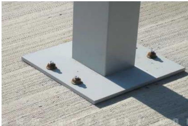
Fastening on a plain concrete pavement
