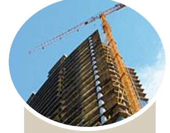
Curtain Wall Facade
