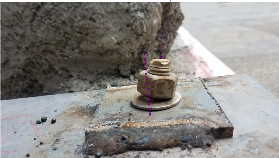
Photo 172.6 View of tilted bolts.
