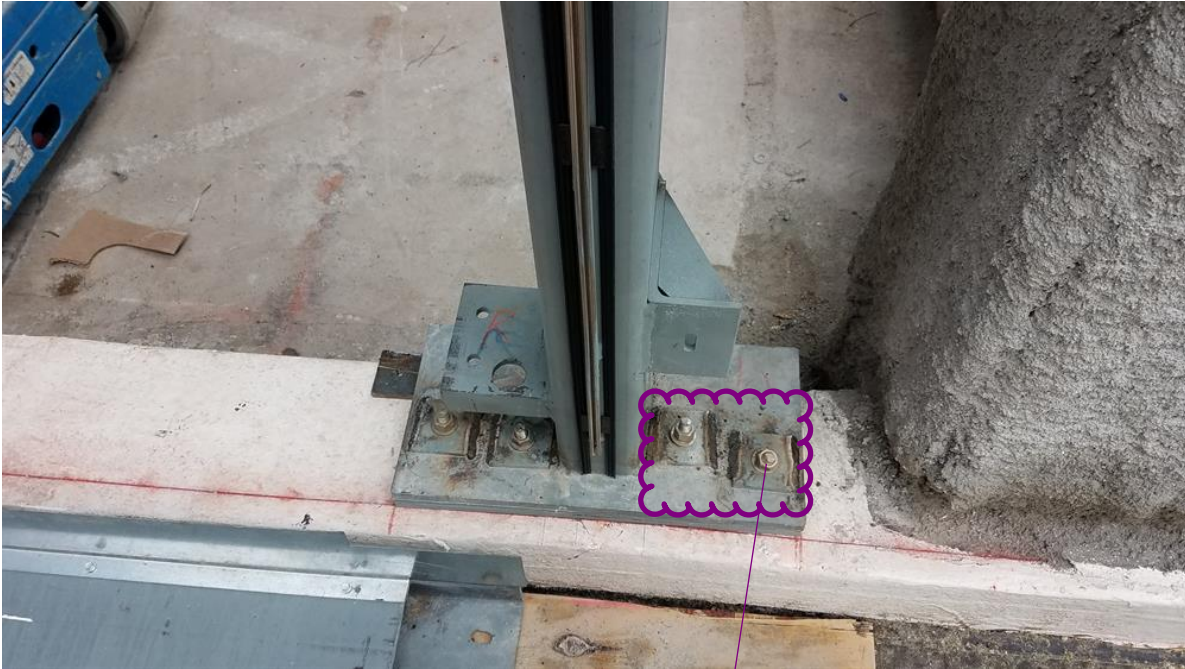
Photo 172.6 View of tilted bolts.
