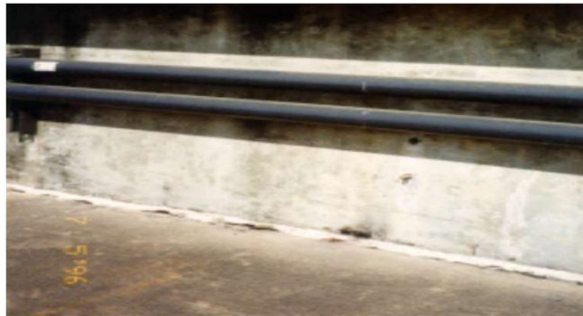
Pipefitting and electrical installations
