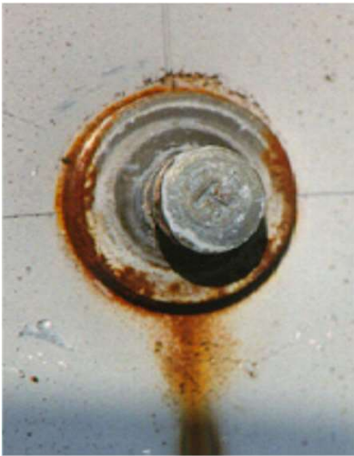
Galvanised nail in an A2 sheet
