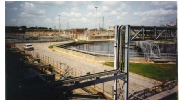
X-CR in a water treatment plant
