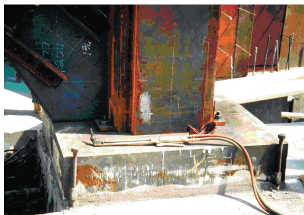
Fig. 2.2. Base plate with adjusting screws.
