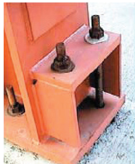
Fig. A1.2. Column moment base using stool.
