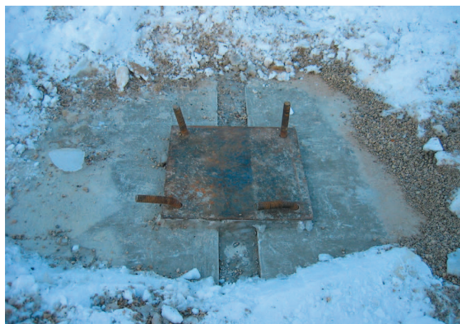
Fig. 2.3. Anchor rods run over by a crane.
