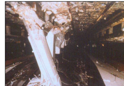
Concrete panels falling from the J.C. Penney store, 1964 Alaska earthquake - 2 people died
