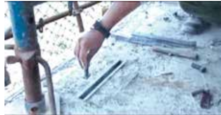
Step 8 – Sliding channel bolt into position
