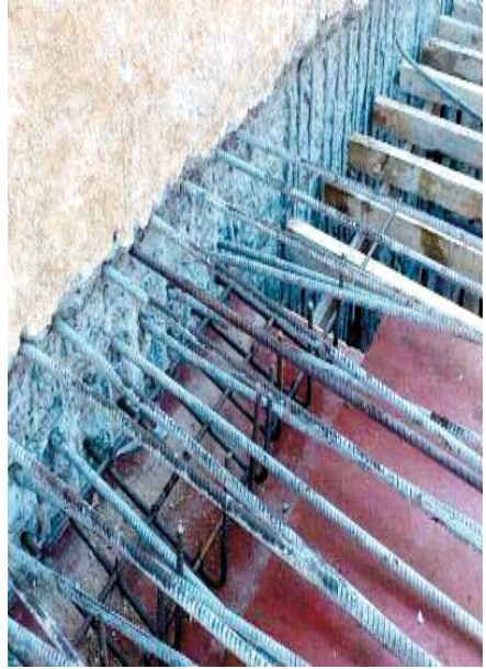
(b) Slab erection from D-Wall
