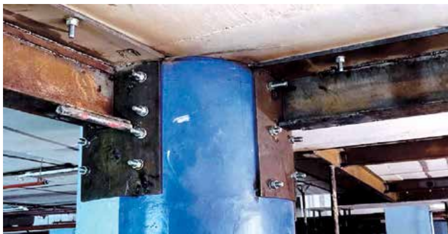
(a) ISMB fixing on column
