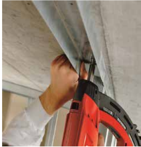
(f) Dry wall track fastening to concrete
