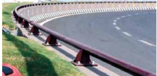
(c) Crash barrier fixing
