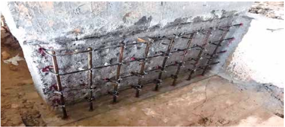
(c) Column strengthening
