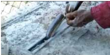
Step 7 – After checking level of channel in hardened concrete, removal of filler material
