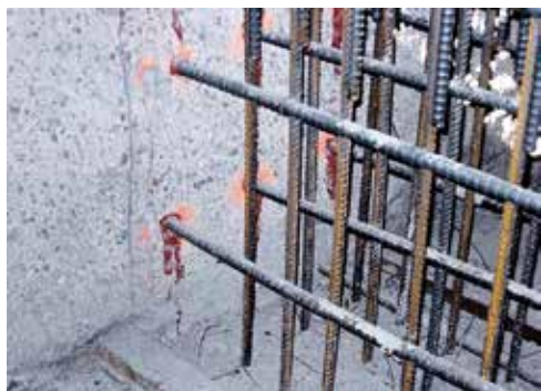
a. Wall-to-wall connection
