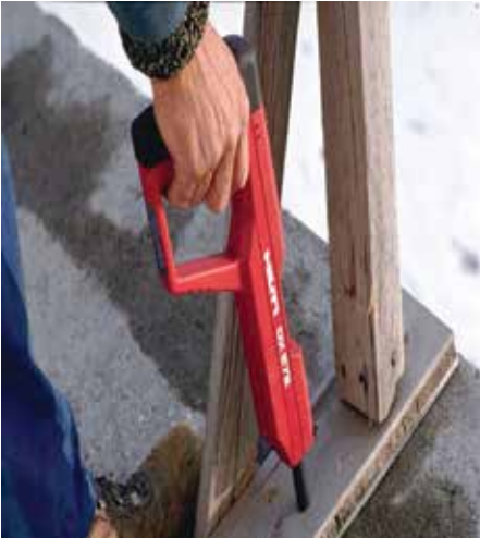
(e) Fastening of wooden batten to concrete
