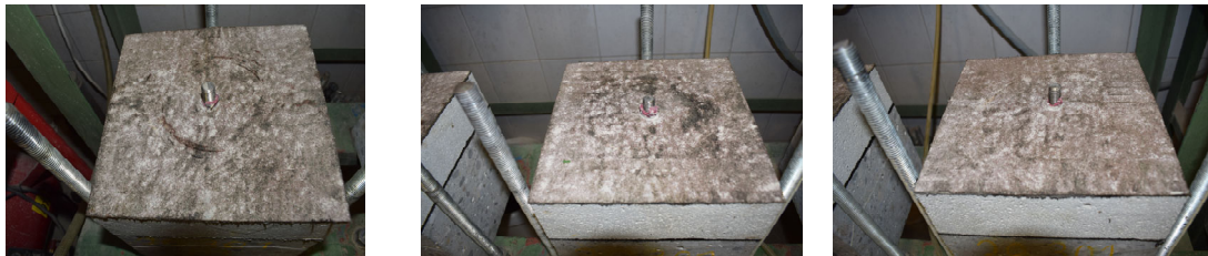
Figure 5. Surfaces of specimens no. 20.301 02 (left), 20.301 03 (middle), and 20.301 04 (right) after removing the ceramic tiles and the tile cement layers.
