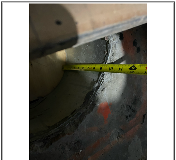
9.5 inch depth of concrete
