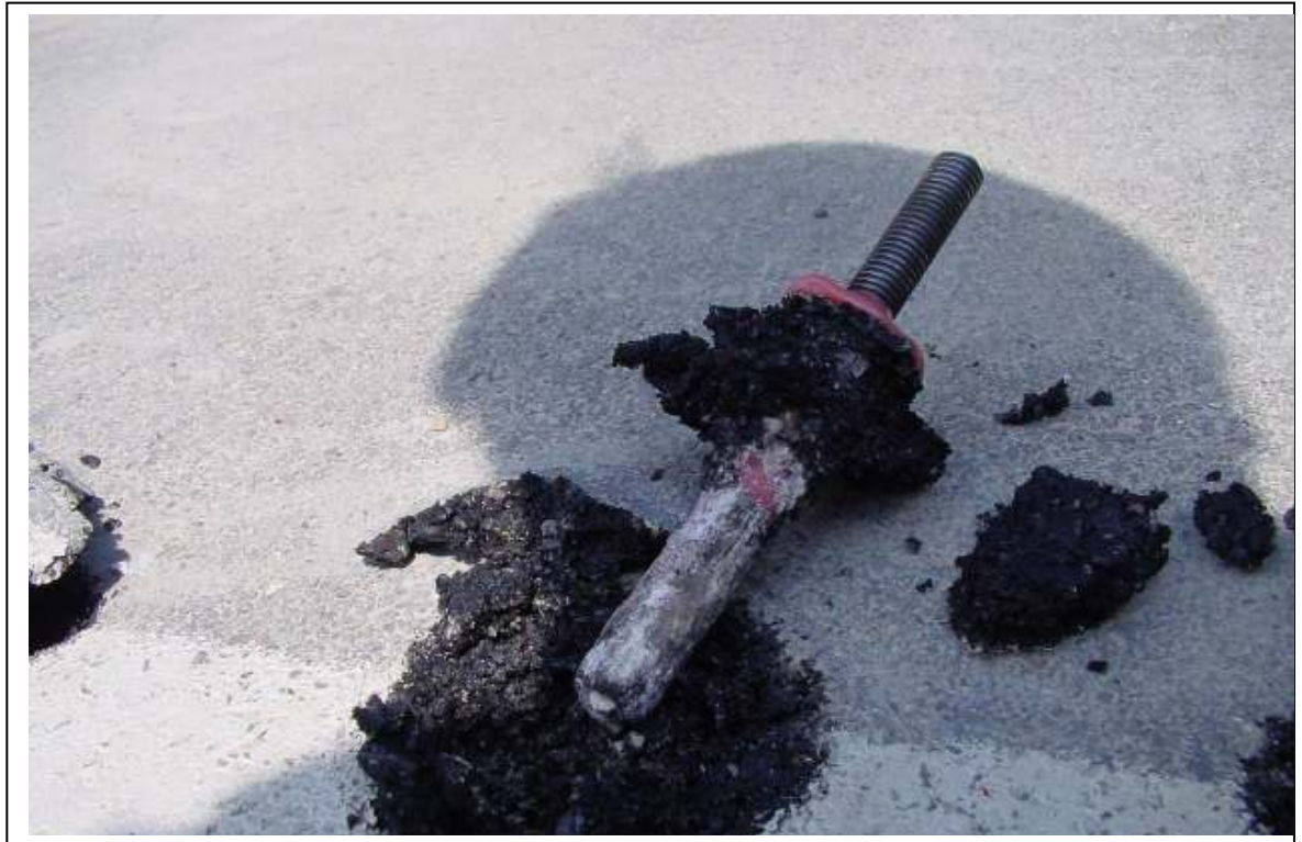
Picture 3: A layer of approx. 1 to 2 mm of asphalt is bonded to the HIT-RE 500 mortar
