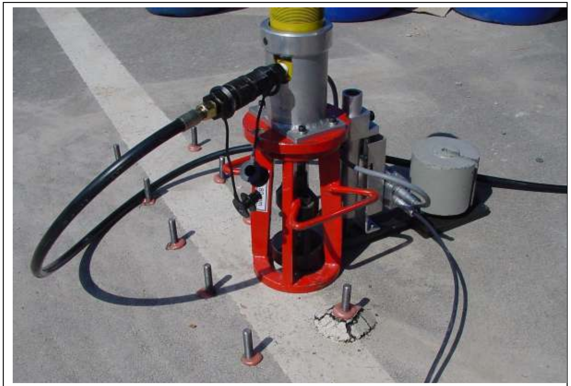
Picture 1: Tension test of anchors HAS M12 fastened with Hilti HIT-RE 500 injection mortar in base material asphalt using the Minipull test equipment.
