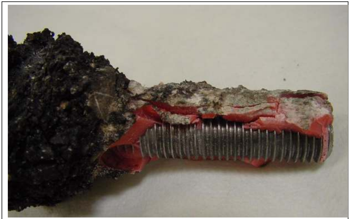
Picture 4: The HIT-RE 500 injection mortar is fully cured and bonded to the asphalt surrounding the mortar.
