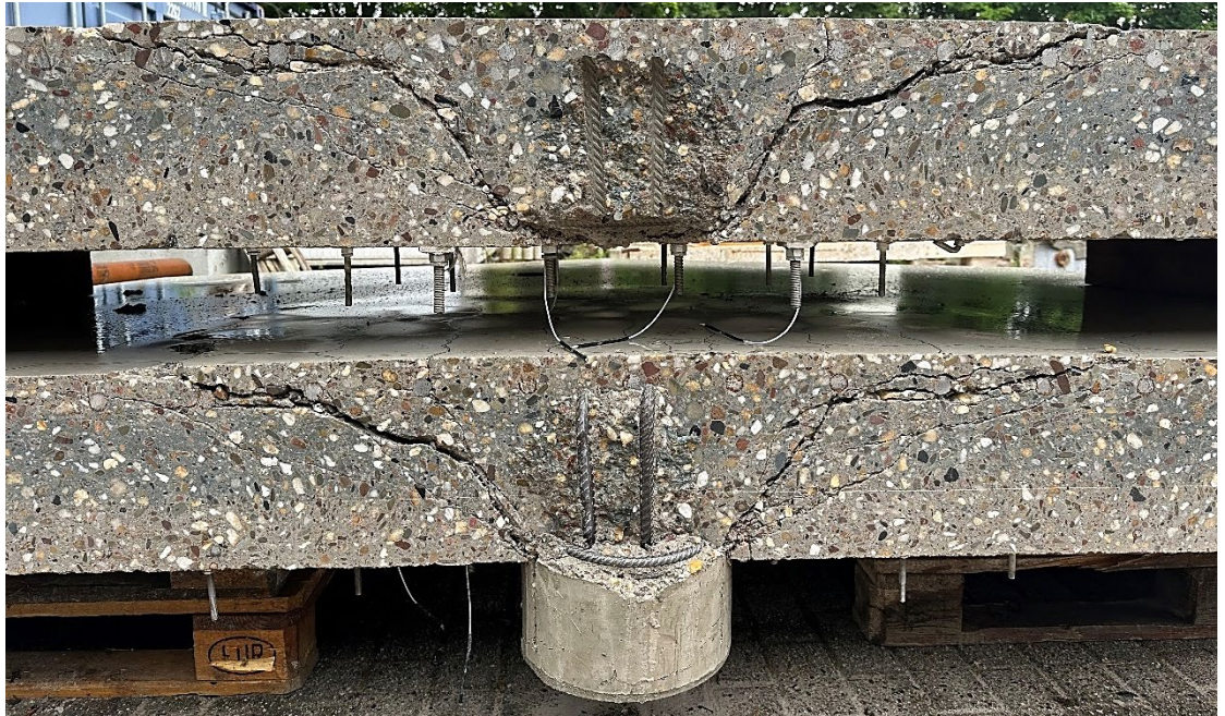
Figure 4: Flat slab specimens highlighting formation of the shear cracks and the truncated cone © Hilti
