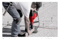
Set the shear connectors using Hilti setting tools featuring TE-C or TE-Y connection ends.
