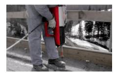
Inject Hilti RE 500 adhesive mortar through the funnel-shaped opening in the shear connector.
