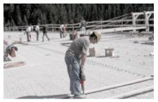
Drill the holes using the Hilti TE 70-AVR rotary hammer and Hilti TE-C3X 16/47 drill bits.
