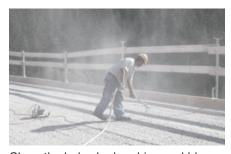
Clean the holes by brushing and blowing out with compressed air using the appropriate Hilti accessories.
